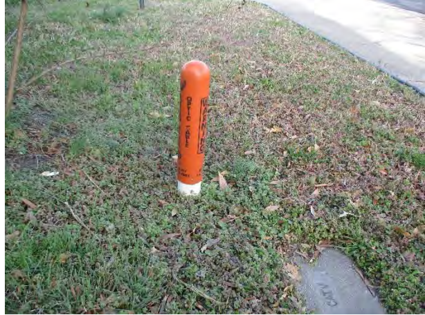
Photograph 14. View of the buried optic cable located in the northwestern portion of the subject Site.
