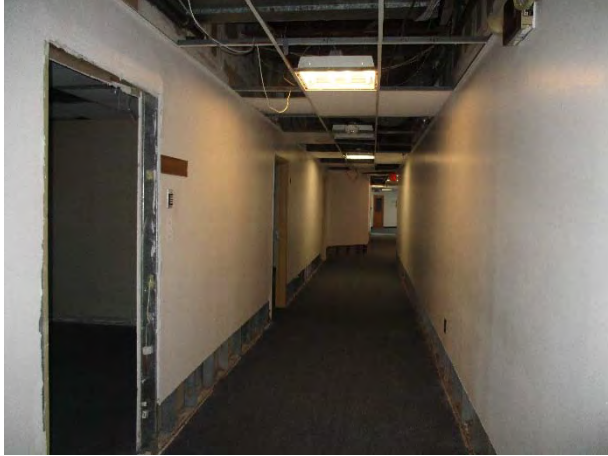
Photograph 25. View of the third floor hallway within the on-site building.
