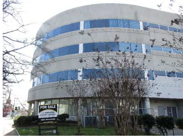
Photograph 2. View of the northern side of the subject Site.
