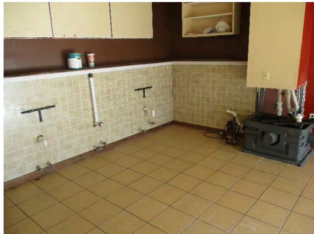
Photograph 24. View of the former kitchen area within the on-site building.
