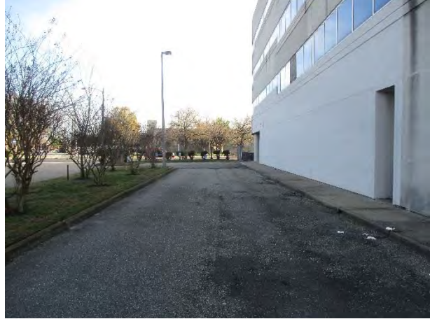
Photograph 6. View of the paved driveway located on the western side of the subject Site.
