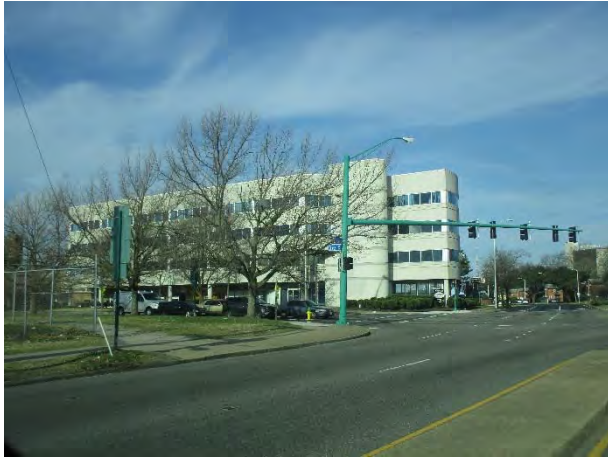
Photograph 1. View of the eastern side of the subject Site.
